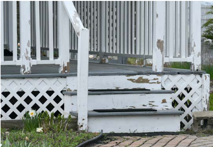
This front porch in Wolfeboro is another example of Blue Jays having peeled and eaten white paint for its calcium content. Photo by Diana Stephens.
