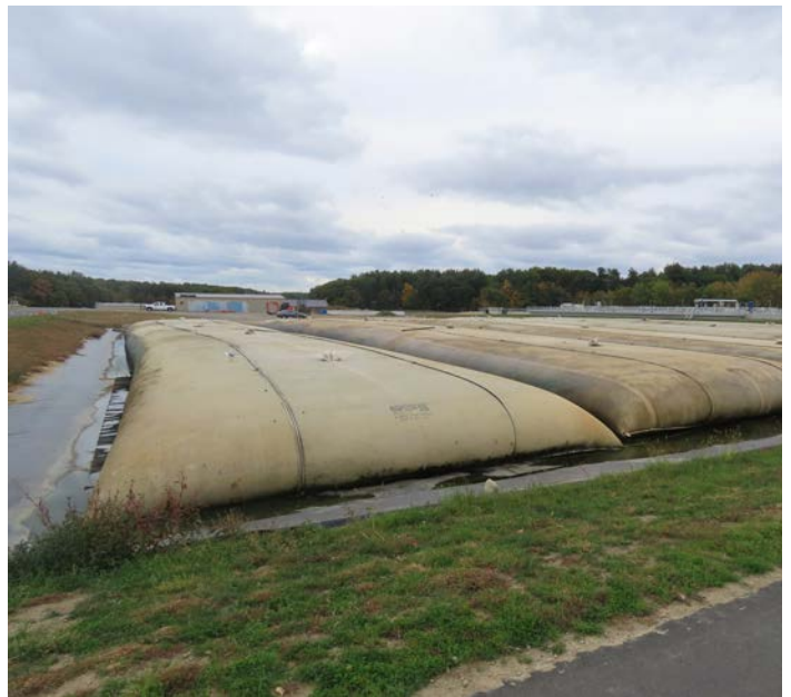
The construction at the Exeter WTP where Lagoon #4 used to be on 9-2-18 (top) and the “pillows” on 10-12-20 (bottom). Photos by Rebecca Suomala.
